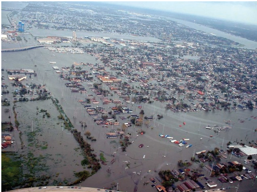
Entire communities, including their supporting infrastructures were washed away.
